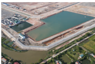
FLOOD PROTECTION DYKE 2
